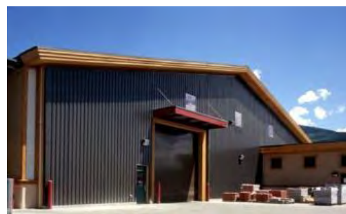
EXHIBIT 4-30: Solar Air Heating System Exterior on a Warehouse
