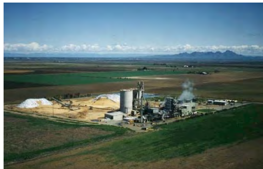
EXHIBIT 3-3: Wadham Energy (Rice Hull-Fired) Direct Combustion Power Plant
