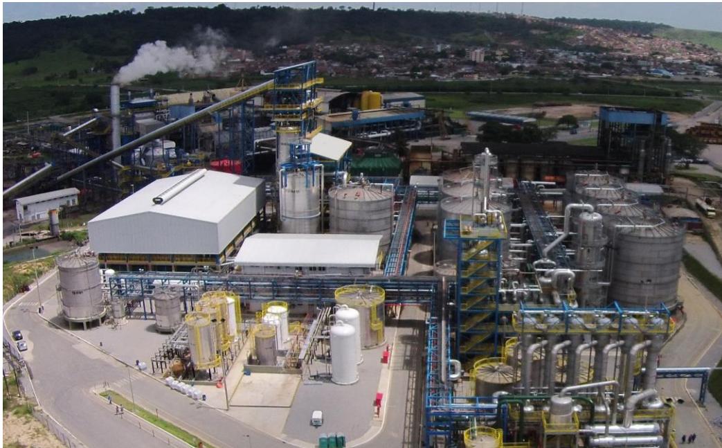
BioFlex I – GranBio’s Cellulosic Ethanol Plant in Alagoas, Brazil
