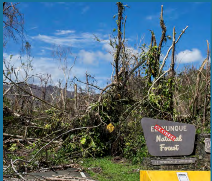
In the aftermath of the hurricanes, El Yunque closed for repairs and restoration work. USDA Forest Service photo.
